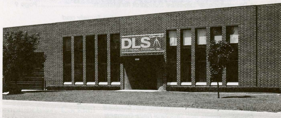
D.L.S.'s new Chicago area EMC test facility in Wheeling, IL
