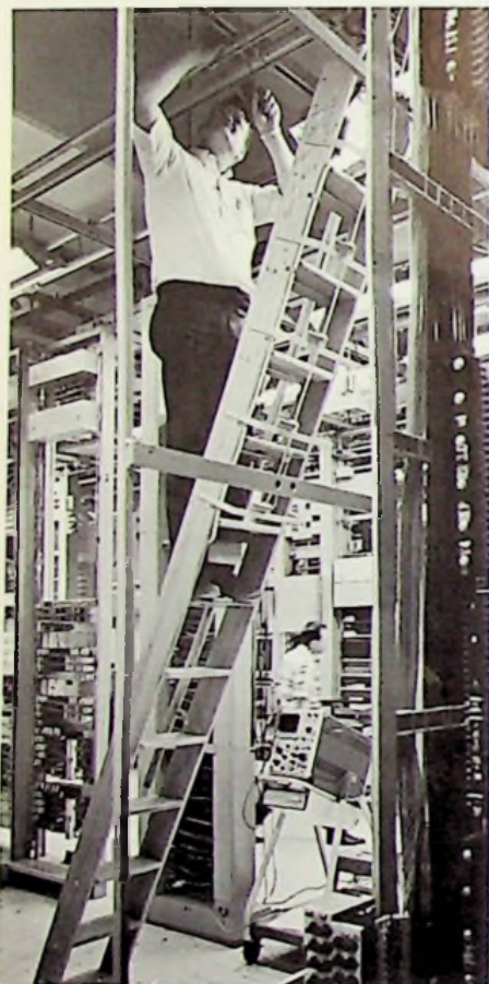
A.T.&T. Long Lines earth link terminal equipment in the earth station at Jamesburg, California in Carmel Valley. This equipment connects overseas satellite circuits to a six-hop microwave system which joins the Bell System's national network in the Bay Area. Workmen in the picture are equipment installers.
