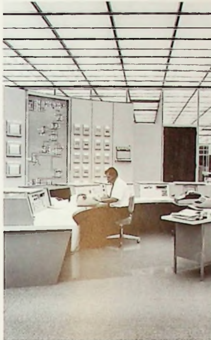
P.G. & E.'s Electric System Dispatch Office at the new Energy Control Center in San Francisco showing the "Power Broker's" Computer Console and Telemetering Display Panel.
