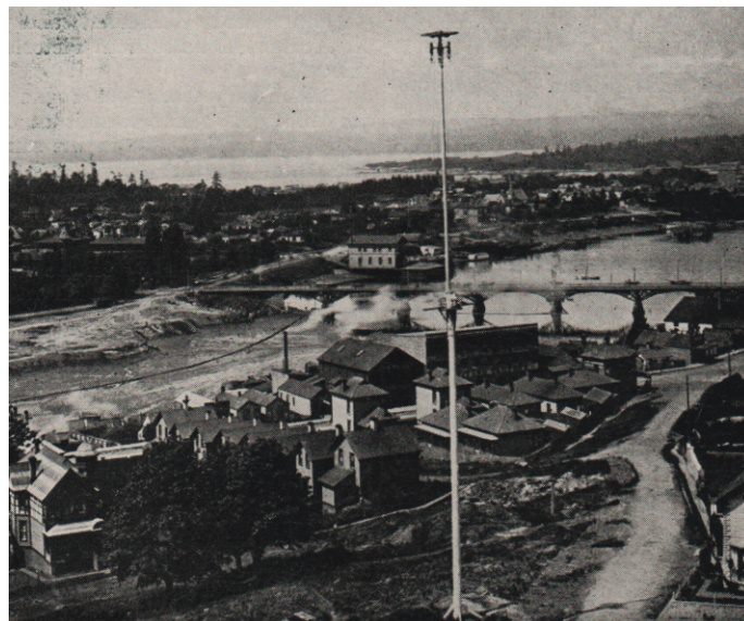
Photo of Early Victoria showing one of the 150 foot lighting masts referred to in this article. Photo courtesy of B.C. Electric Railway Company.
