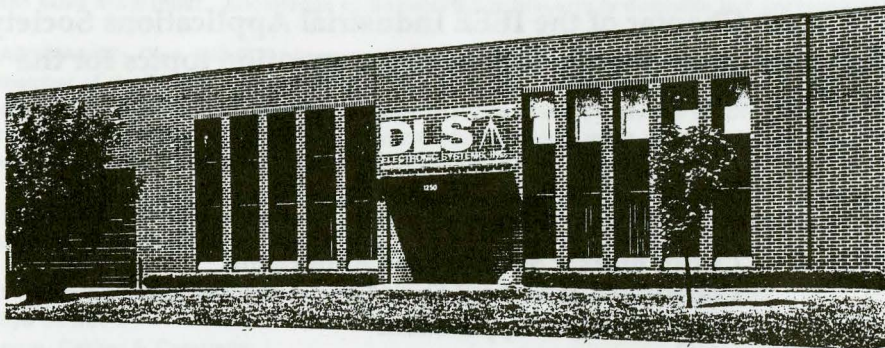
D.L.S.'s new Chicago area EMC test facility in Wheeling, IL
