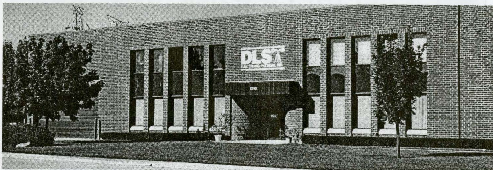
DLS's new Chicago area EMC test facility in Wheeling, IL
