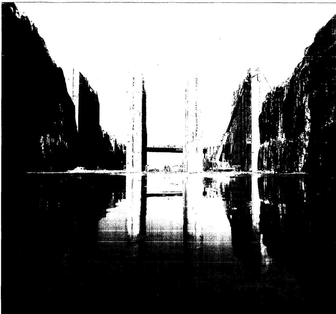
Construction—Eastmain River, James Bay Power Project. Photo courtesy of Hydro-Québec.
