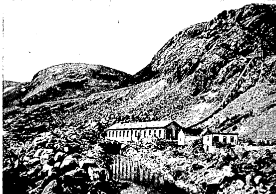
Power house, penstock and flume, Petty Harbour Hydro Electric Development, Newfoundland—1900. Photo courtesy of Newfoundland Light and Power Company.
