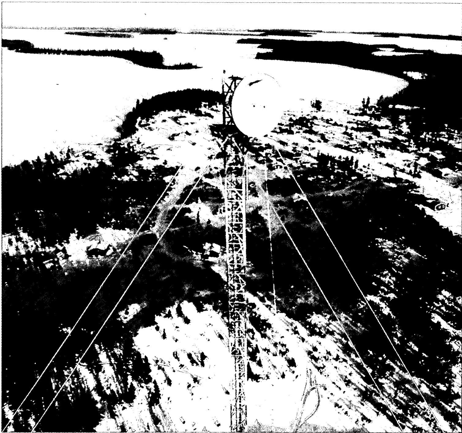
Microwave tower provides telephone and television services to remote areas of Northern Ontario. Photo courtesy of Bell Canada Telephone Historical Collection.
