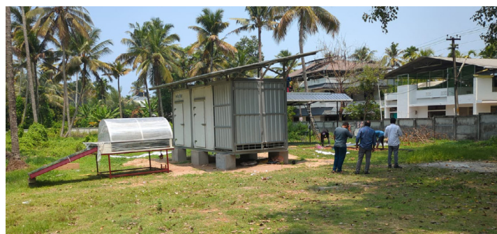
CRE Hub's solar dryer and solar-powered cold storage equipment during installation.
